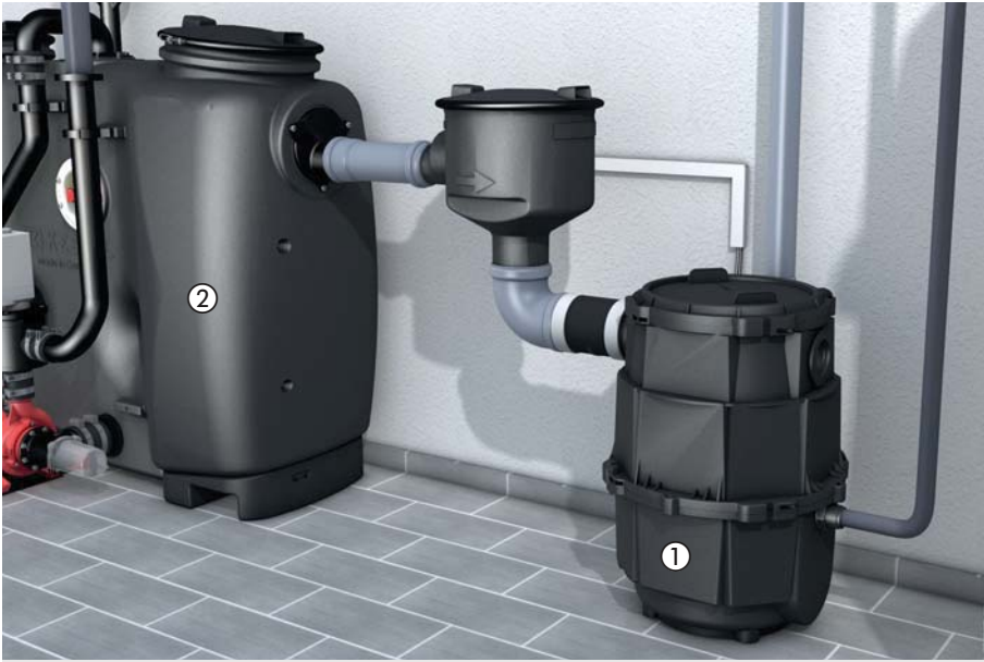
① Lifting station Aqualift S ② Grease separator EasyClean
