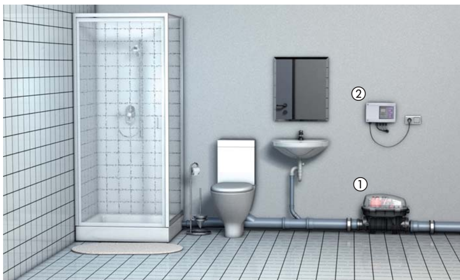
① Backwater pumping station ② Control unit
